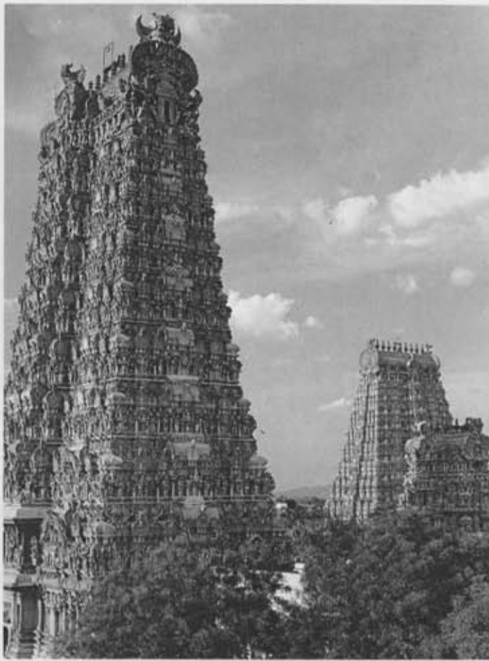
The large Hindu temples are breathtaking buildings. This gate-tower or gopuram leads into the temple of Minakshi at Madurai. Minakshi is a consort of the god Shiva.
